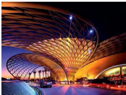
Fig. 1. A triangulated grid-shell structure can assume freeform shapes and require no cable bracing
