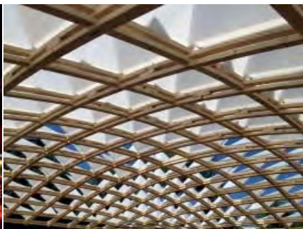
Fig. 2. UTSA Gridshell prototype at the McNay Art Museum
